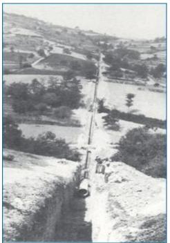
Figure 30 - Picture portraying the laying of one of the main water pipes [62]
